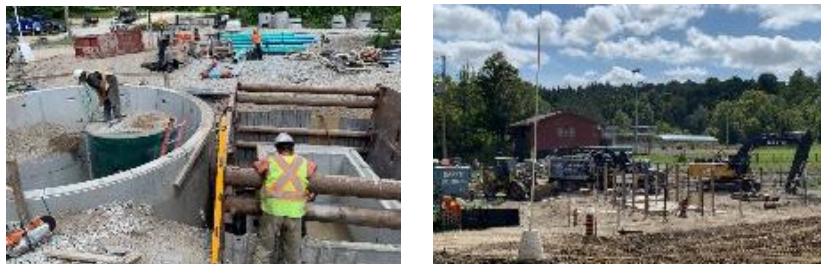
(From top to bottom) Conceptual rendering of Accessible Pool. Architectural Renderings of the Recreational Hall. Site photos during installation of the pumping station for the sanitary service and water main.
