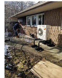
Indian Line air source heat pump as part of the energy efficiency retrofit program
