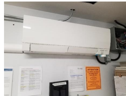
Indian Line air source heat pump as part of the energy efficiency retrofit program
